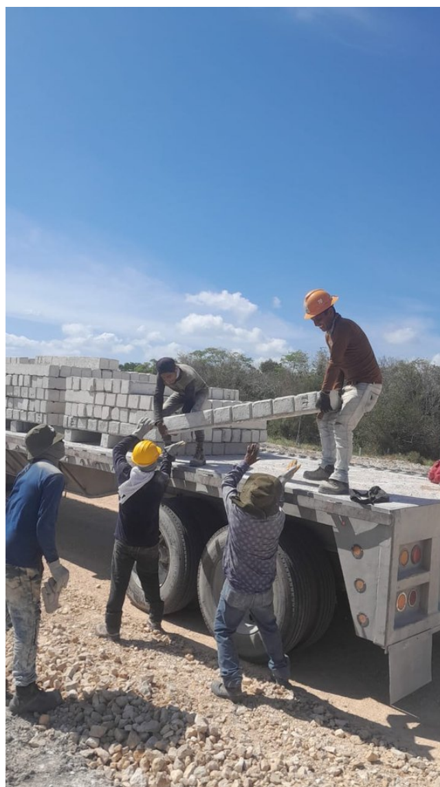
Unloading posts at the work front.
